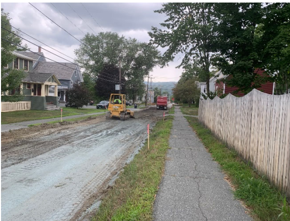
Fine grading of Dana Street
