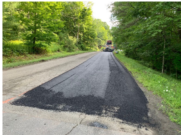
Asphalt leveling course on Brook Road
