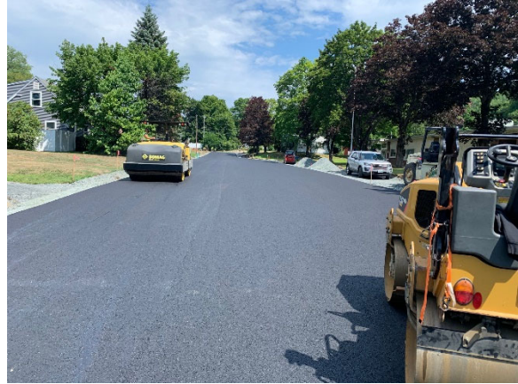
Base pavement installed on White Ave
