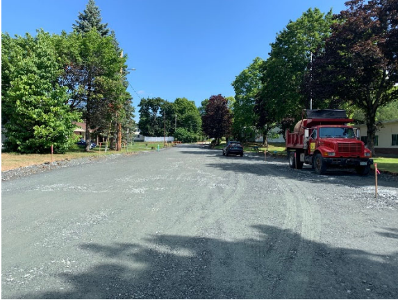
New gravel base for White Avenue
