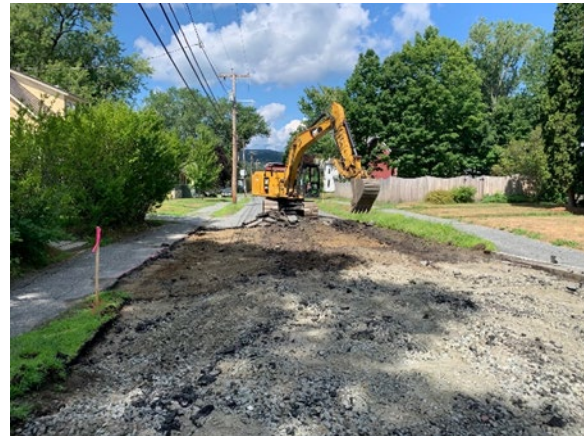
Pavement Removal on Dana Street
