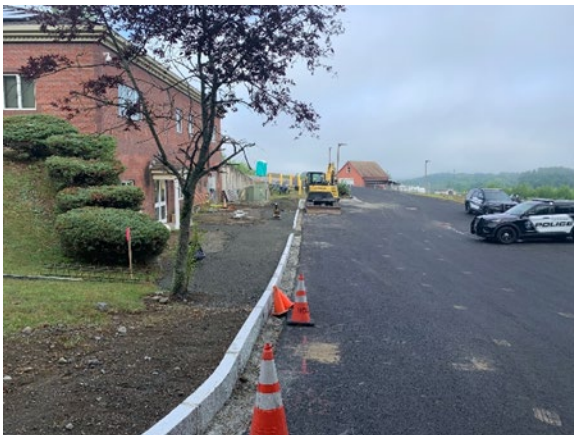
Curb Installation at the Police Dept.
