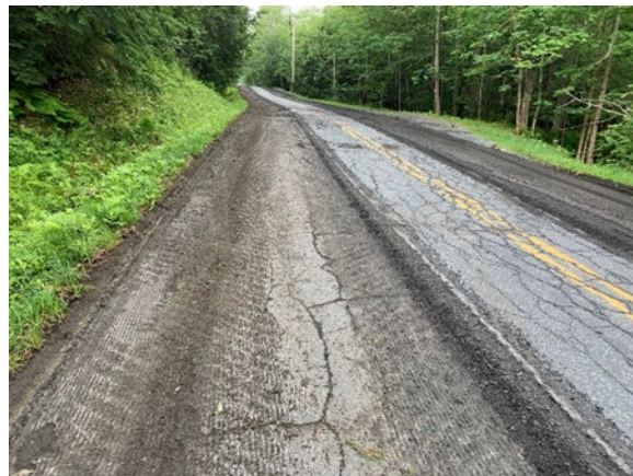
Profile Milling on Brook Road
