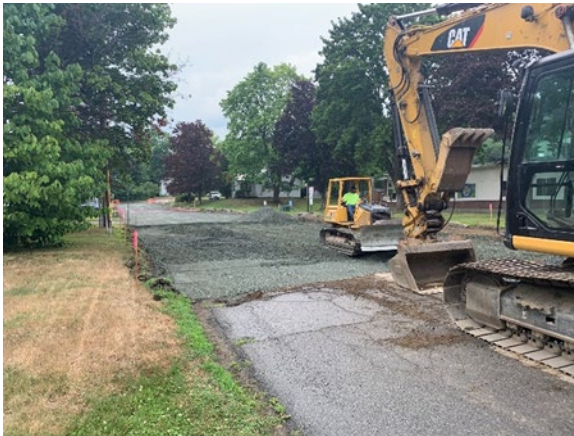
Gravel Installation on White Avenue
