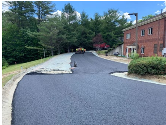
Paving base on the North side
