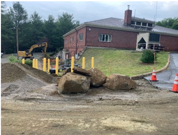
Site preparation work
