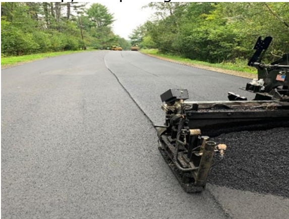
Blacktop, Inc. paving Moss Road
