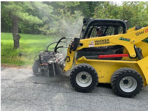
City Highway crew removing pavement for shoulder & future savings.
