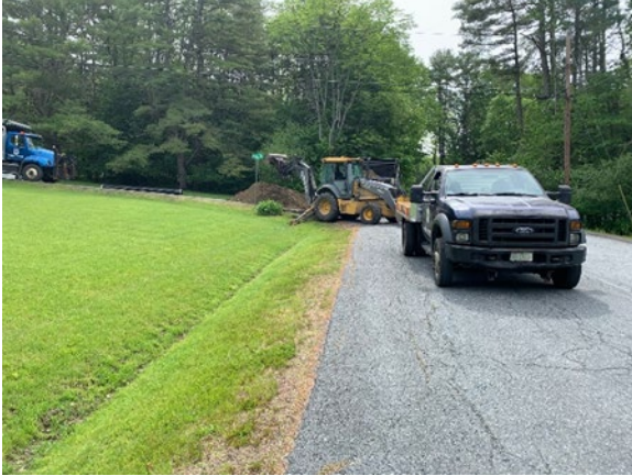
City crew installing culvert, Moss Rd
