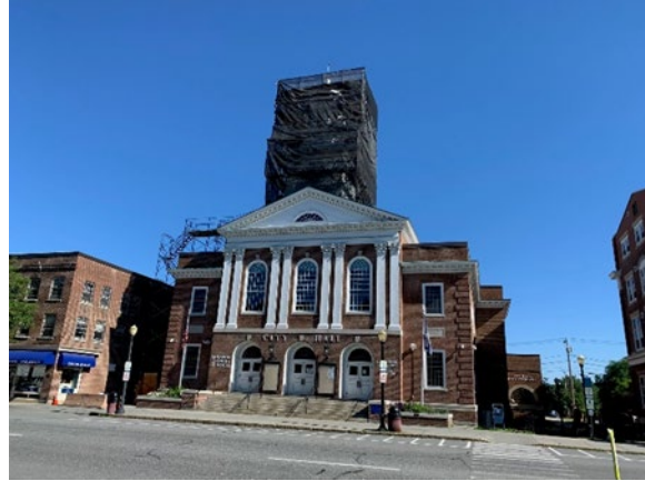
City Hall tower painting begins
