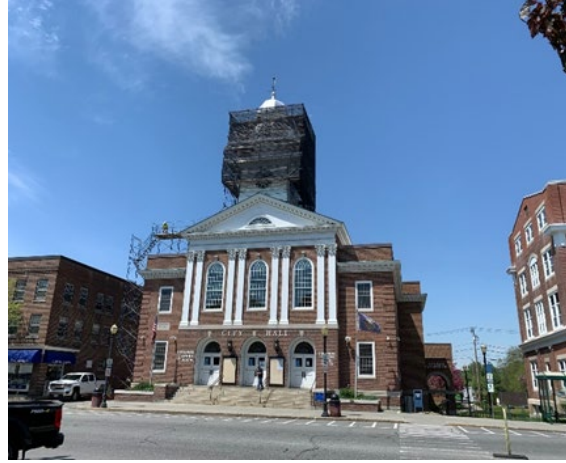
L&M topsoiling around Colburn Park. Scaffolding being installed for painting.
