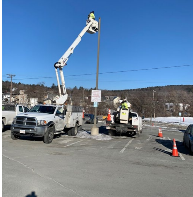
Pineridge Technologies installing a new LED streetlight behind City Hall
